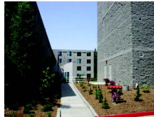
Azusa Pacific University: Building materials
