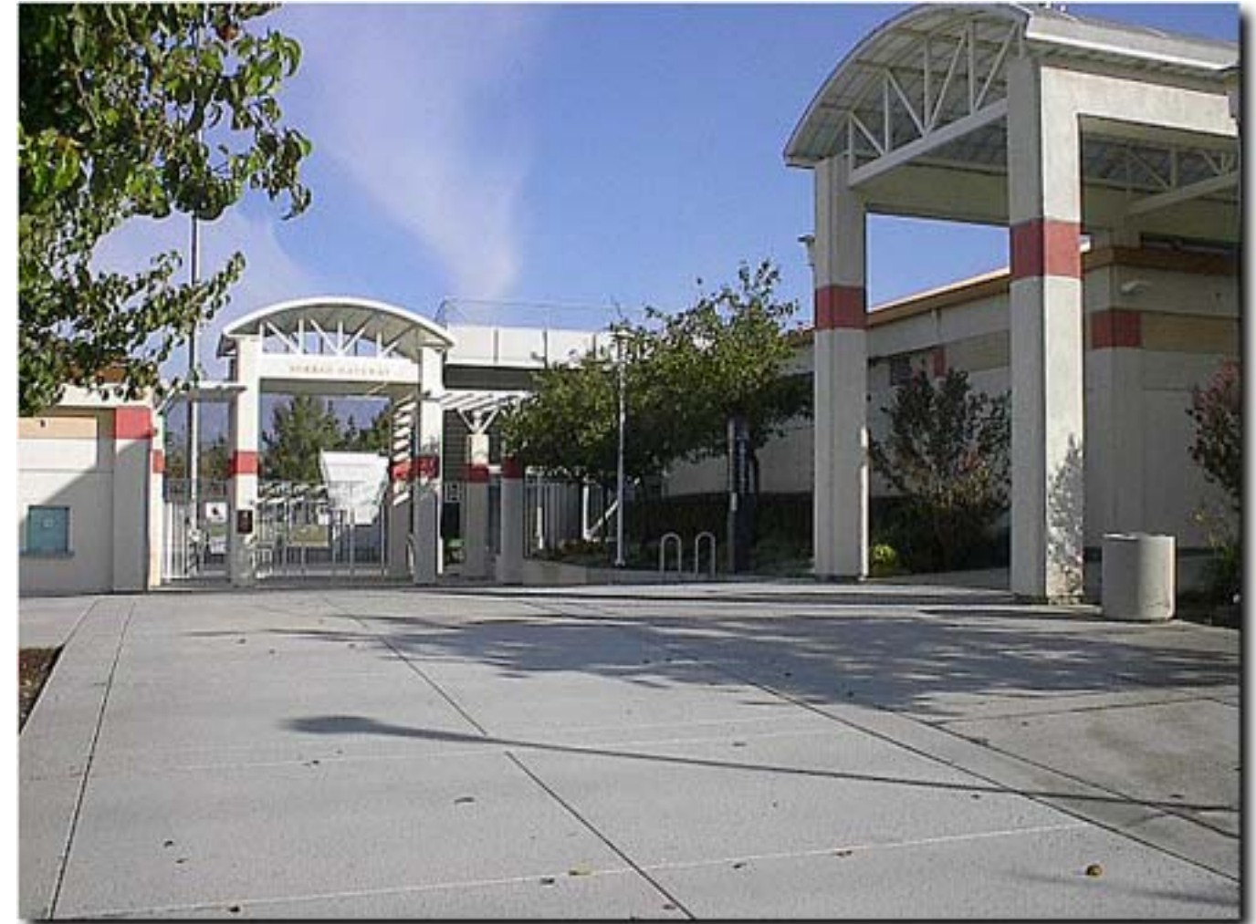
University of Redlands: Entry to physical education facilities
