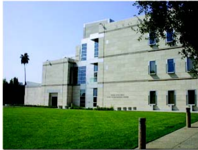
California Institute of Technology: Roof elements
