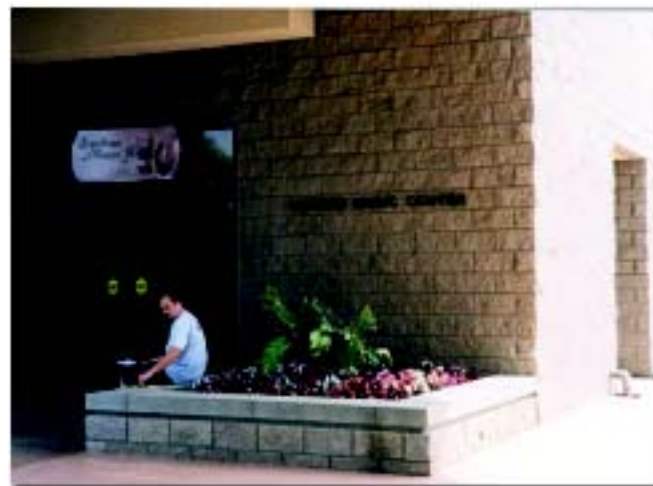
Azusa Pacific University: Building entrance
